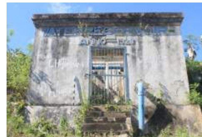
Gambar 4. Bangunan Water Reservoir Anno 1928 (Sumber: Dok. Penulis, 2016)
